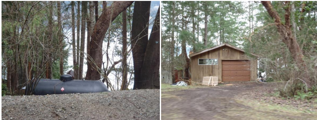
Figure 13. Propane tank adjacent to central ring road (left), structure with surrounding vegetation within 10 m (right)
