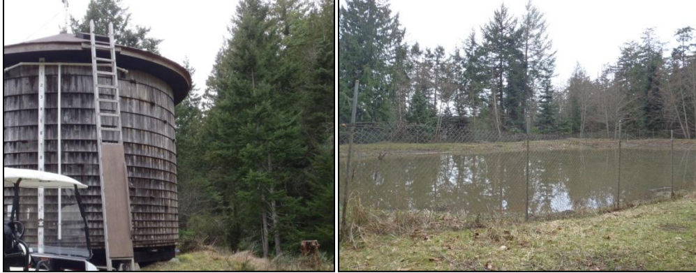
Figure 3. Water tower and central reservoir.
