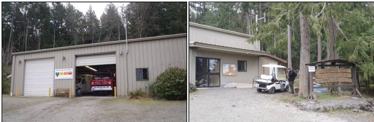
Figure 2. Piers Island Fire Hall.
