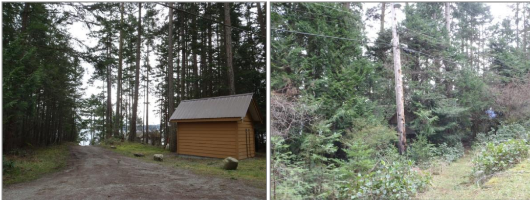
Figure 5. Pumphouse for municipal water (left) and wood distribution poles for power and telephone (right).
